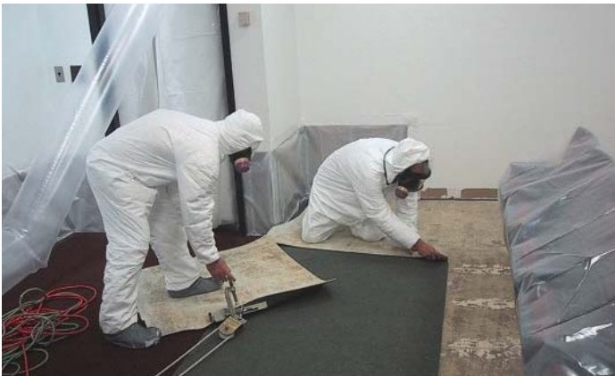
Carpet removal behind protective enclosure.
