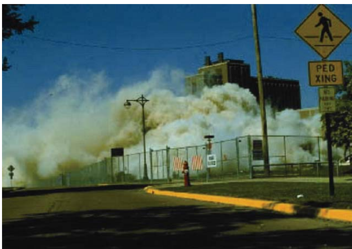
Demolition of adjacent structure.
